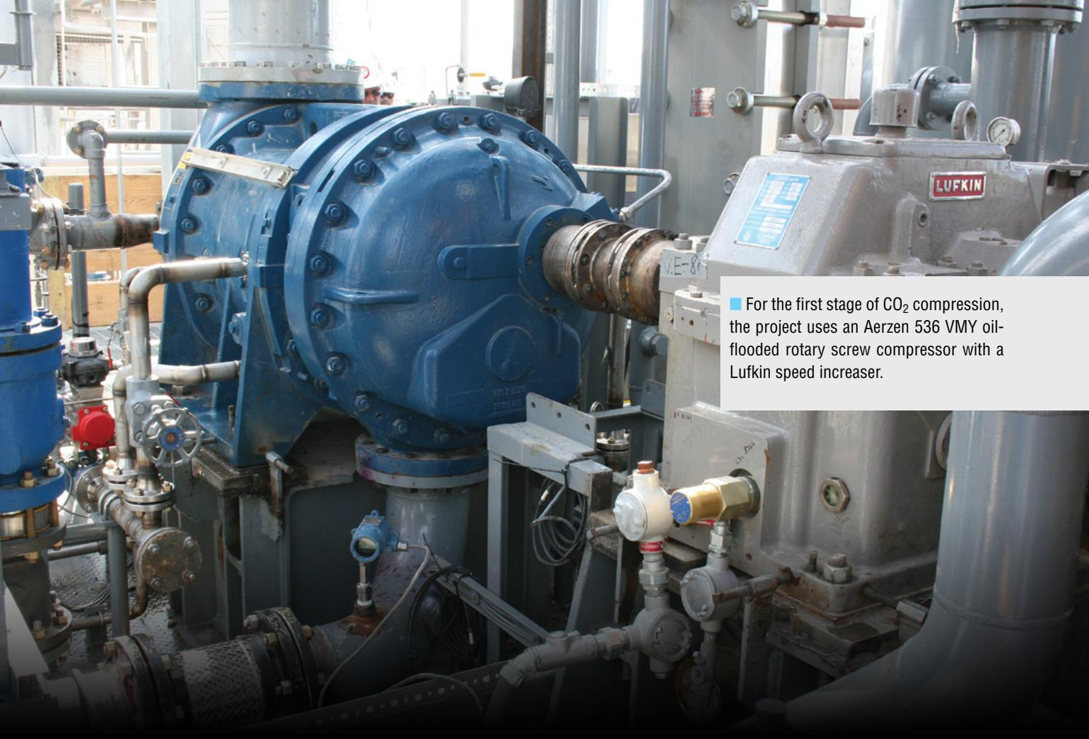
■ For the first stage of CO<sub>2</sub> compression, the project uses an Aerzen 536 VMY oil-flooded rotary screw compressor with a Lufkin speed increaser.
