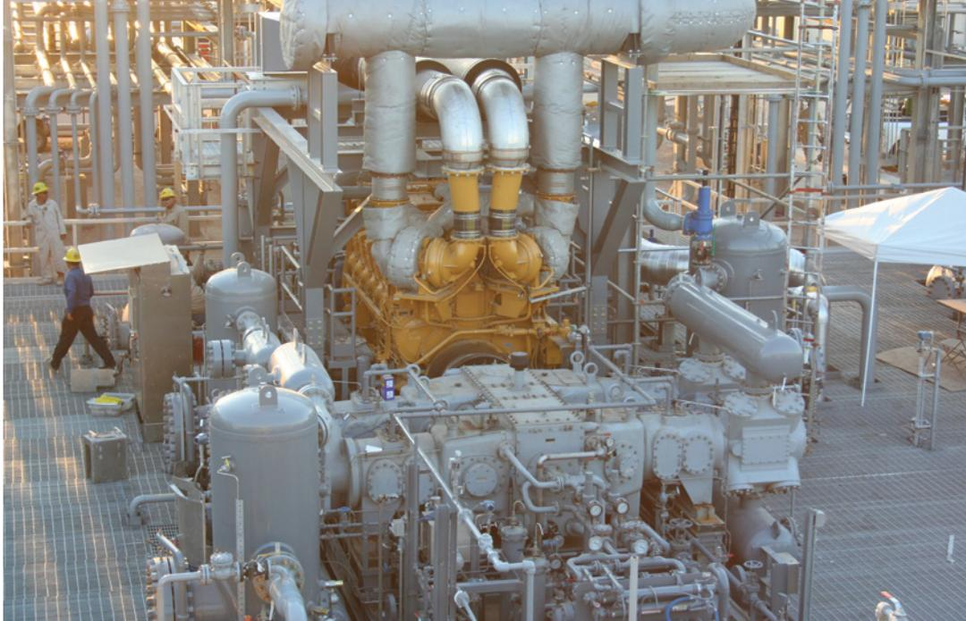
■ For the second through fourth stages, the project uses a Neuman & Esser 3 SVL 320hs reciprocating compressor driven by a Caterpillar G3612 TA natural gas engine.
